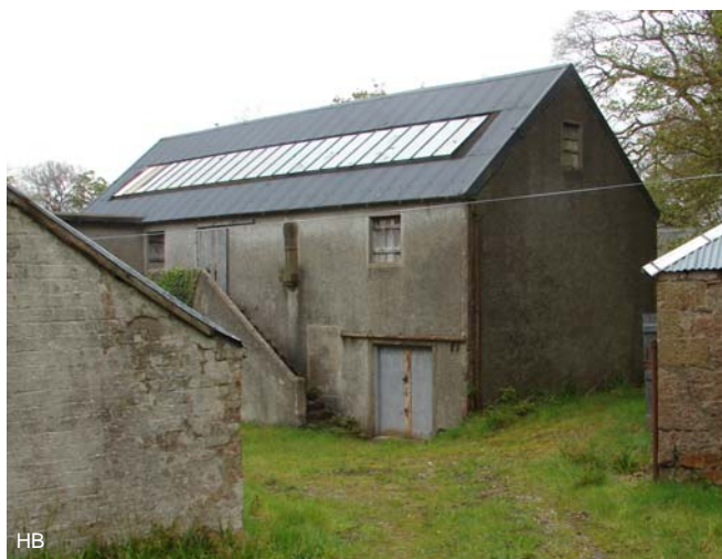
Against the wall below it is an external stone stair, which still gives access to the workspace.
