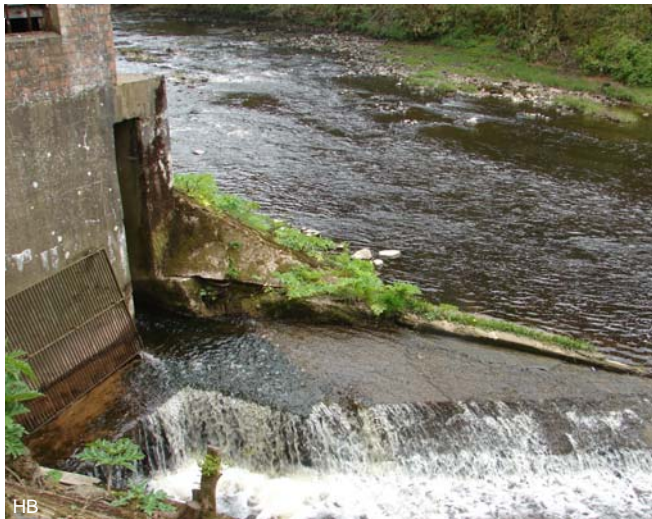
Outlet of the generator at the Milton mill.
