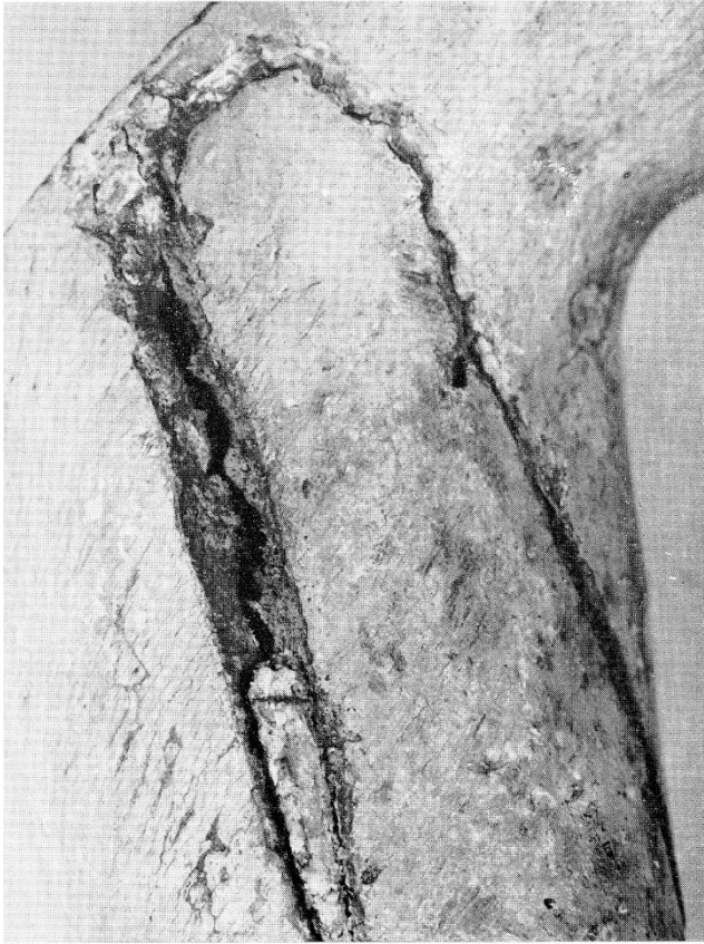
FIG. 6 - The left forearm. The filler in the gap between two pieces of wood partly disintegrated. (Photo: Nordic center for restoration in Florence).
