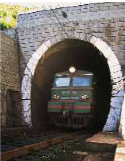
Photo1. Entrance Beskyd tunnel
