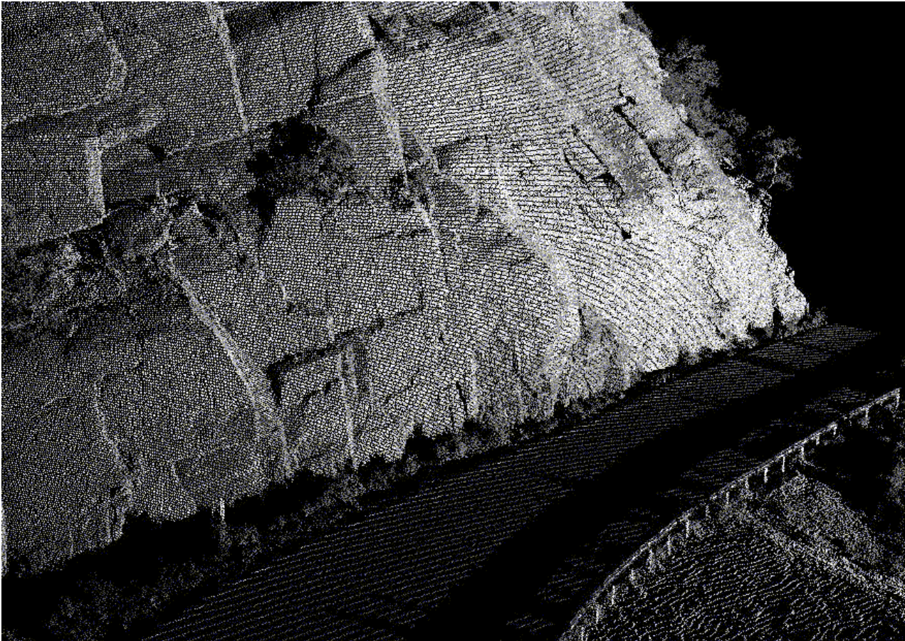
Figure 1. A typical point cloud representation of a highway rock cut. Visible rock cut is about 10 meters high.
