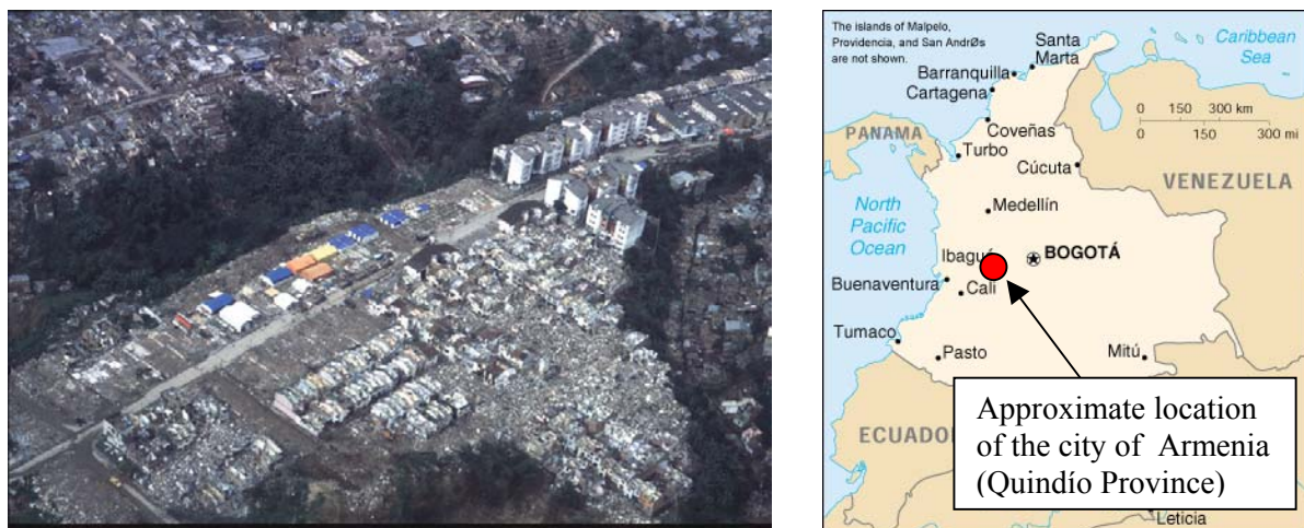
Figure 1. An area in Armenia, that was severely damaged by the earthquake
