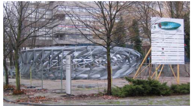
Figure 18. The steel structure of the iWeb building at TU Delft.
