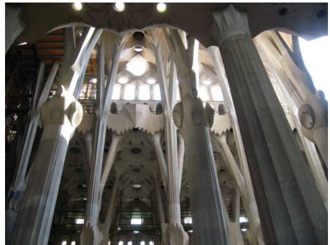
Figure 5. Roof support structure of the central nave of Gaudí's Sagrada Família church.
